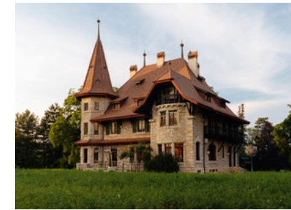
M.A.D House Exterior view
